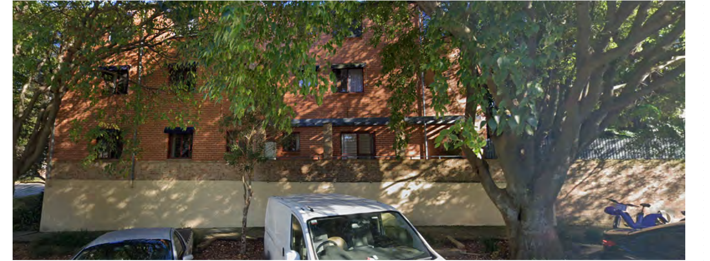
2 Kensington Mews - Morehead Street frontage
